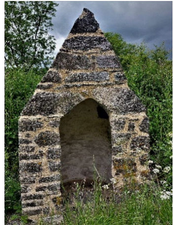
Yealmbridge Toll hut front (Photos: Tim Jenkinson)
