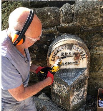
Paint removal in progress
