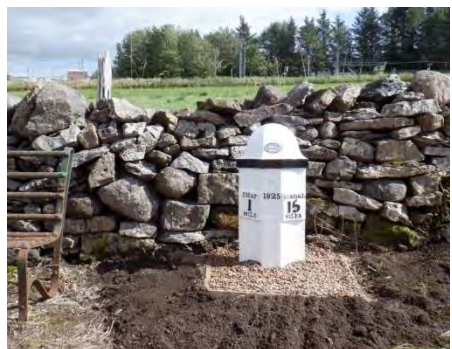
CU_PRAP01 after restoration
