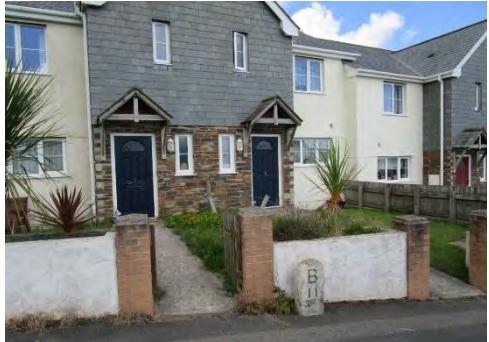
Grade II listed milestone at SW925595 in front of new houses at Indian Queens
