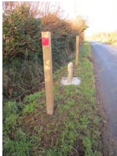
Newquay 6 at SW8755 5696 A3058 repaired, reinstated, protected Photo: Ian Thompson
