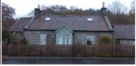
Roadman's Cottage (Hillend) Photo: John Riddell
