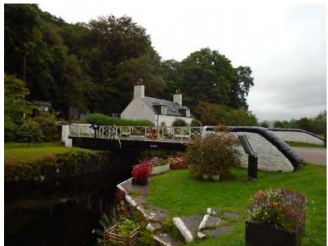
Crinan Canal bridge and cottage
