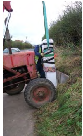
Broughton Cross milestone restoration
