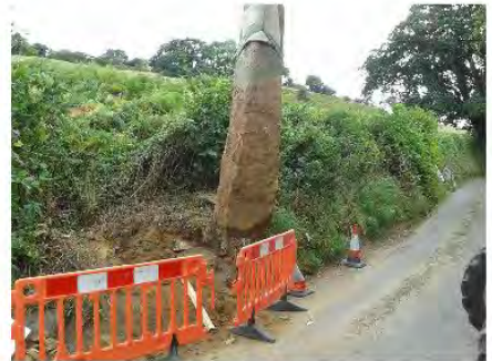
The Stone proved to be longer than expected; This required a hoist to lift it out.
