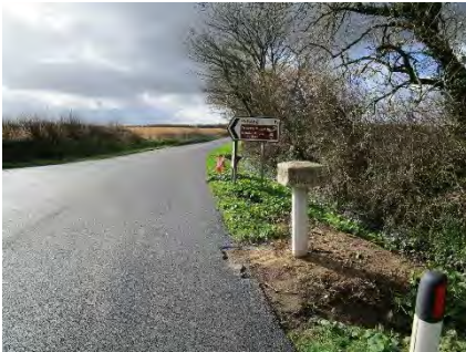
SX05785 72124 B3266 St Mabyn 67733 relocated with new column 7.3.19
