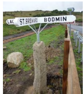
SX136736 A30 Temple overbridge with restored granite fingerpost August 2018 Photo: Ian Thompson
