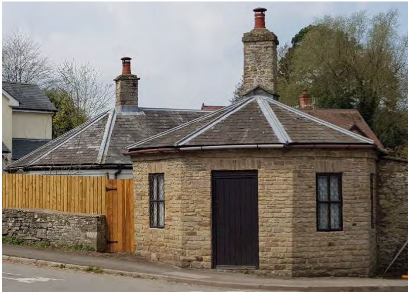
The restored Kingswood toll gate in Kington, one of five surviving in the town.
