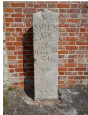
Repaired milestone Photos: Peter Banks
