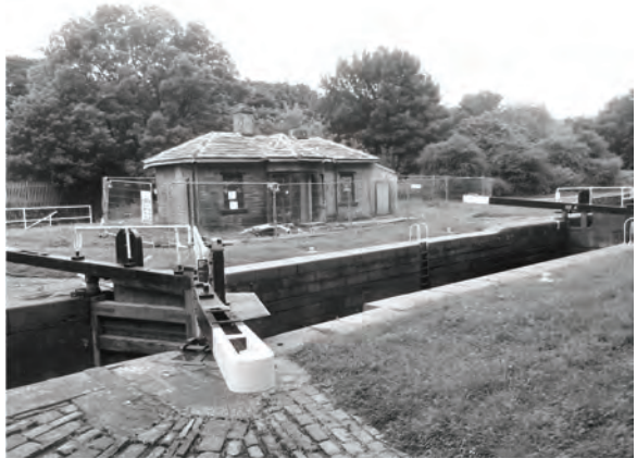
Lock keeper's cottage under renovation
