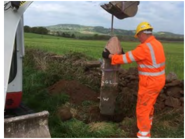
WE_PRAP 03 WHINFELL backing stone insertion
